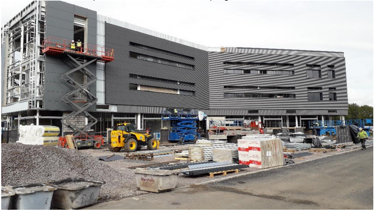
Dock Grow-on Workspace: Exterior construction progress
