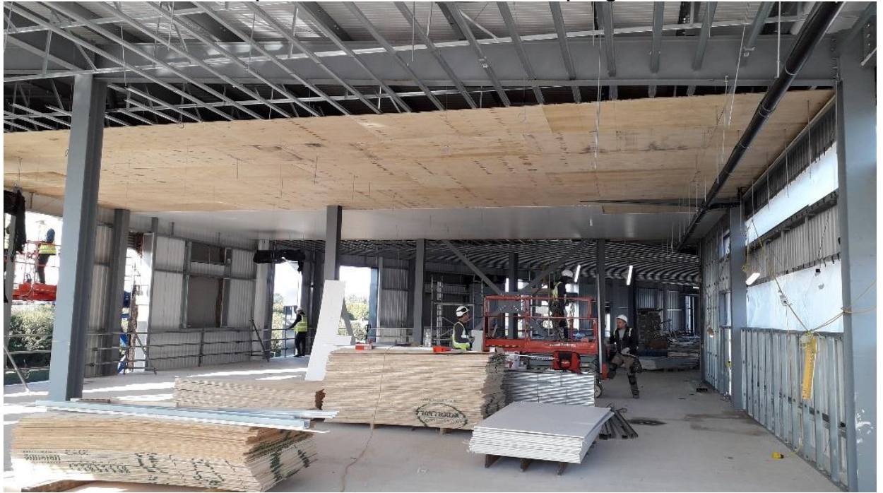
Dock Grow-on Workspace: Interior construction progress
